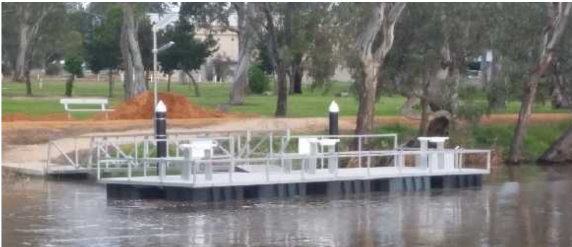
Fishing pontoon at Dimboola, similar to what is proposed for installation at Nhill Lake
