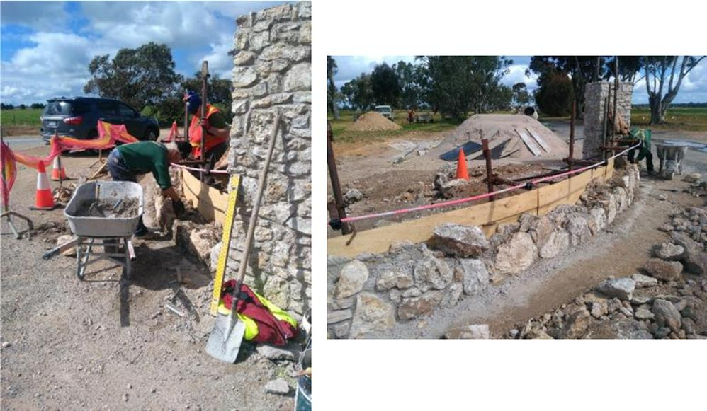
The first photograph shows a worker in a green shirt and safety vest using a shovel to work on a stone wall. A wheelbarrow filled with concrete is in the foreground. The second photograph shows a wider view of the stone wall under construction, with a wooden formwork structure and a pile of stones nearby. |
