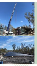
The construction of the new Albacutya Bridge is nearing completion with concrete deck installation being completed recently and works on the road approaches are due to begin soon.
