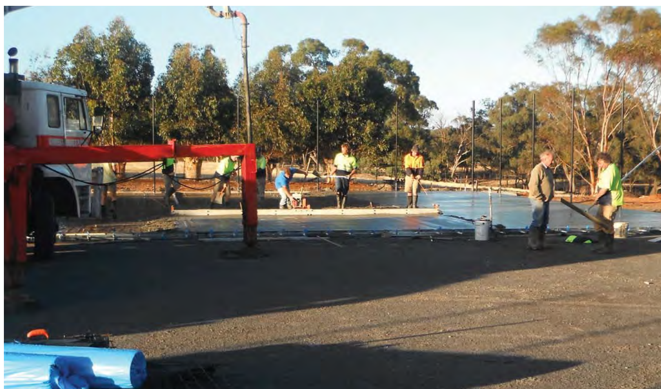
► Pouring concrete during construction of the Antwerp tennis courts
