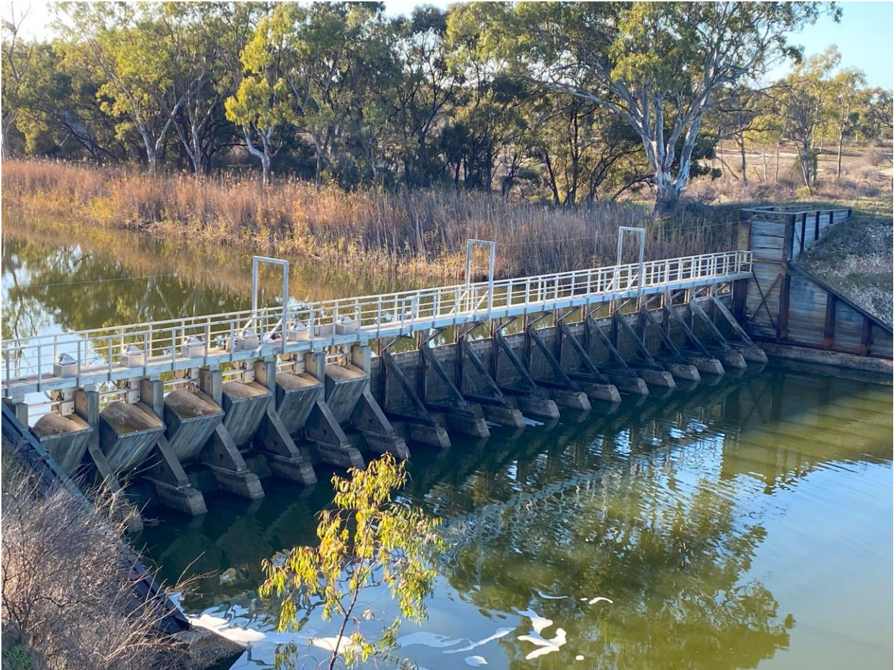
Photograph 1 – General downstream of the weir
