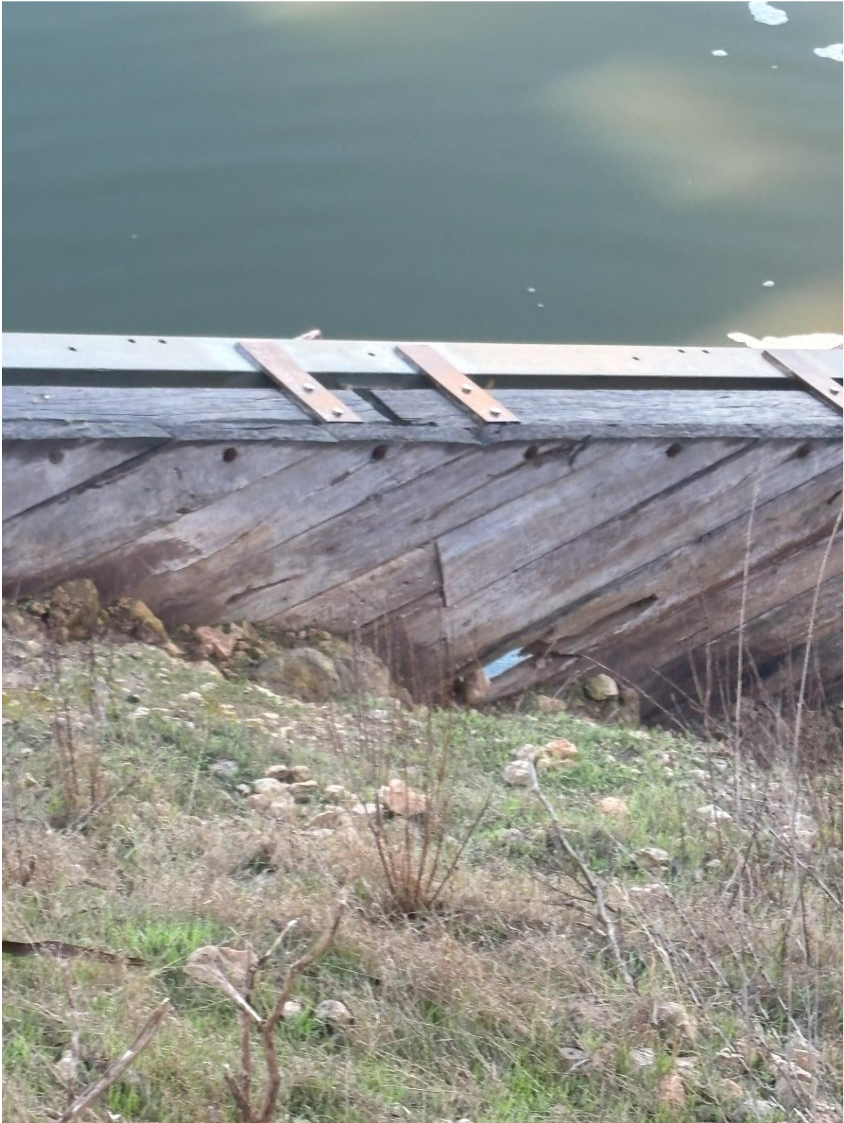
Photograph 14 – Right side retaining wall.
