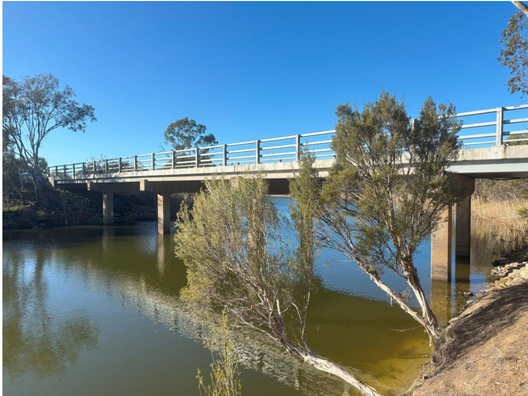
Photograph 20 – Nhill-Jeparit Road bridge.
