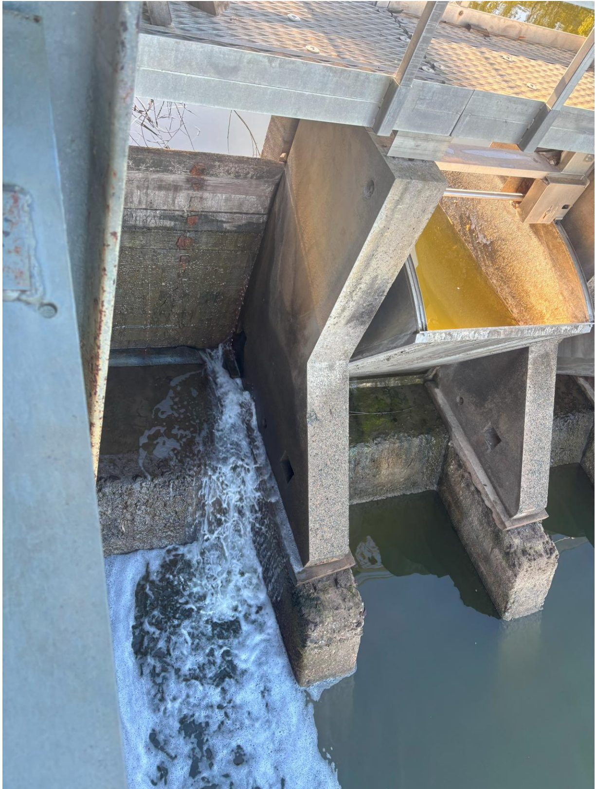
Photograph 17 – Right most bay.
