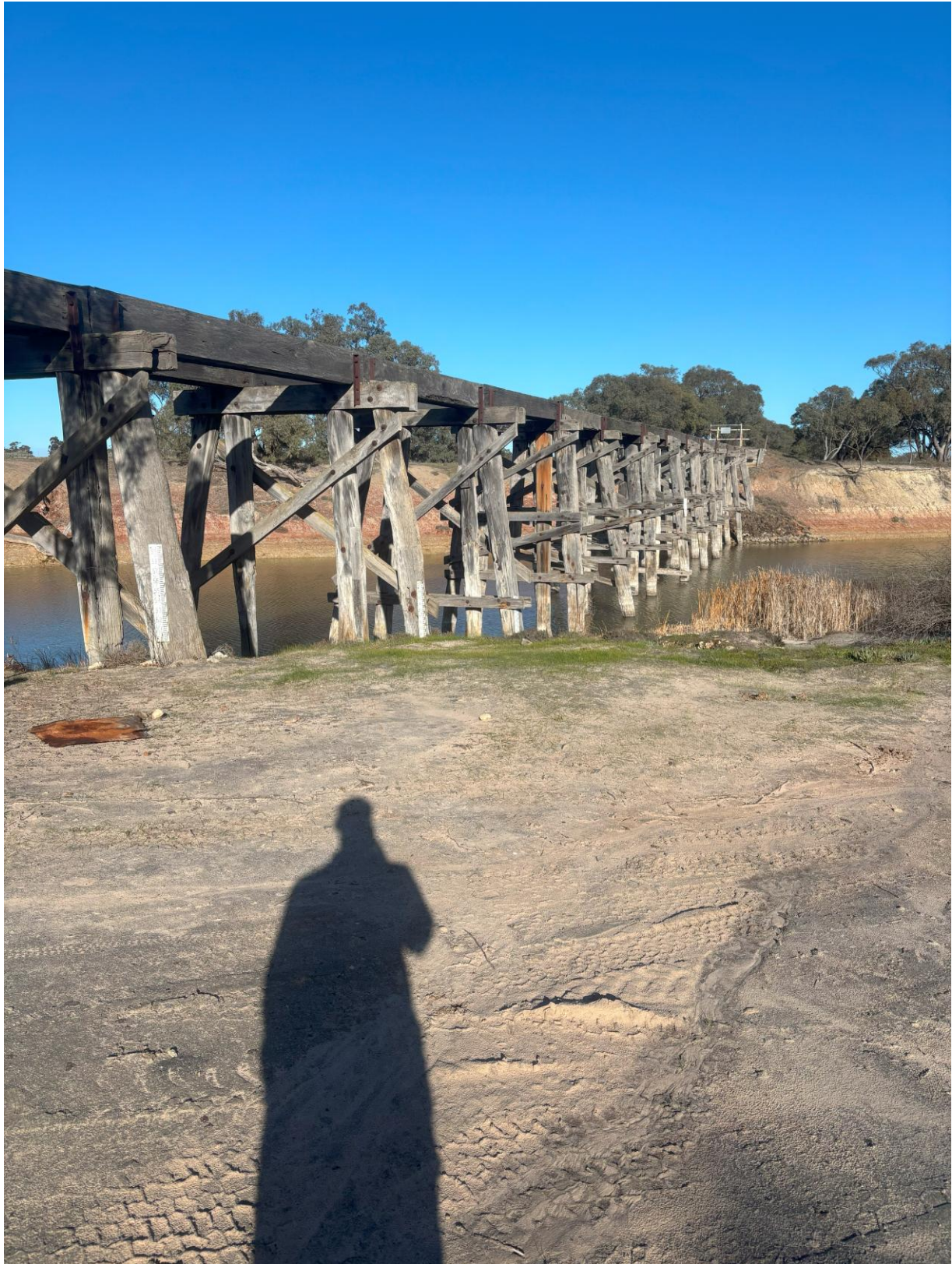
Photograph 18 – Old rail bridge.
