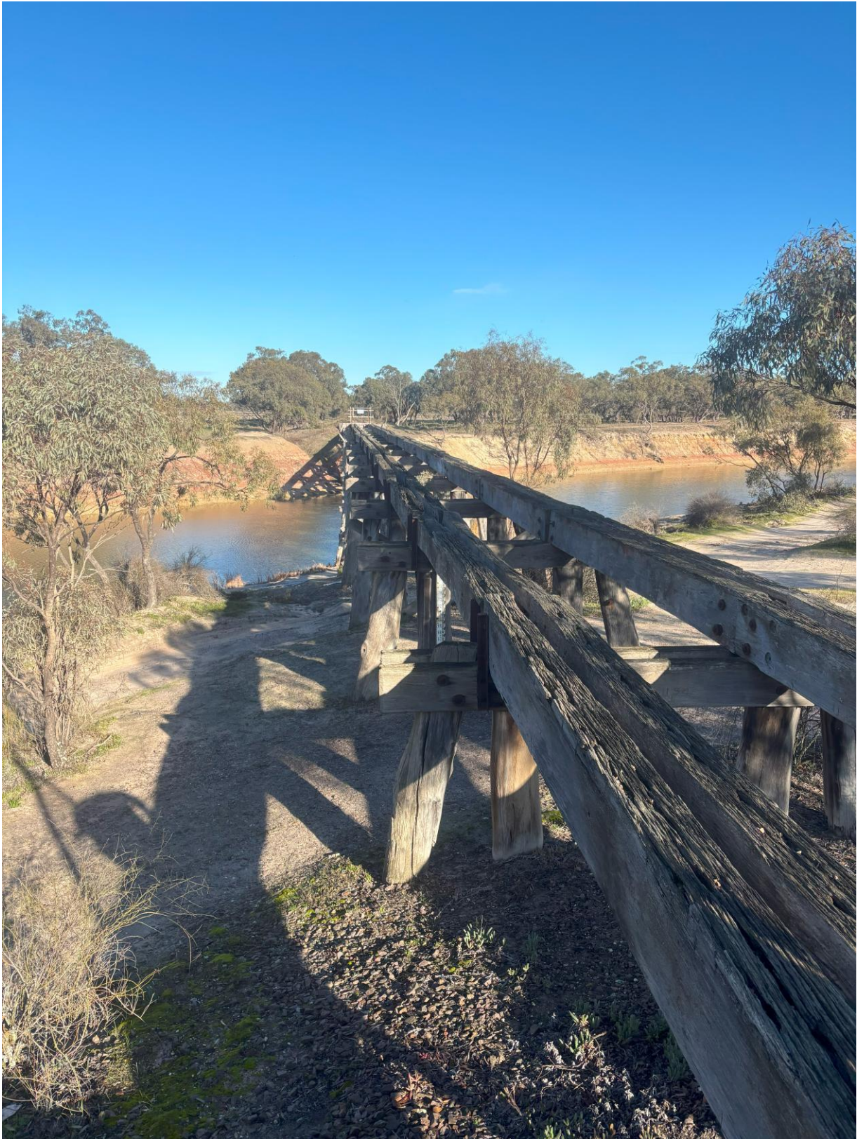
Photograph 19 – Old rail bridge.
