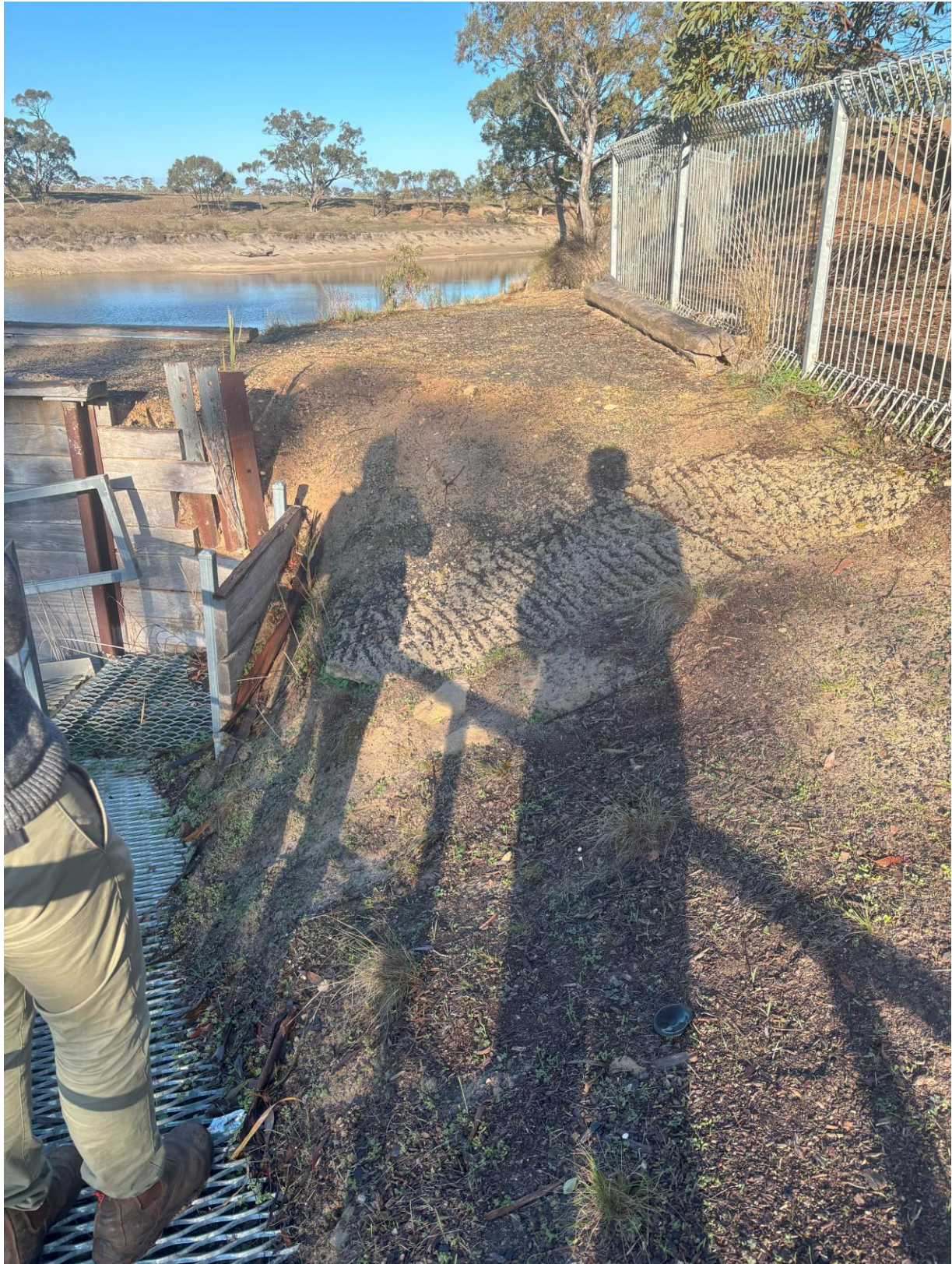
Photograph 11 – Right abutment and retaining wall.
