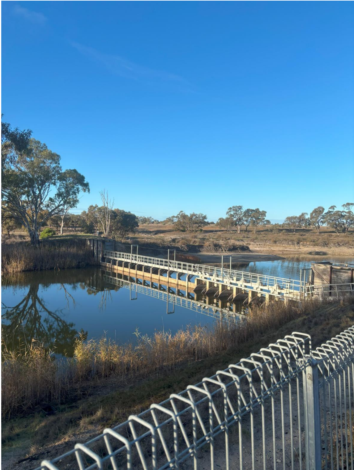
Photograph 2 – General upstream of the weir
