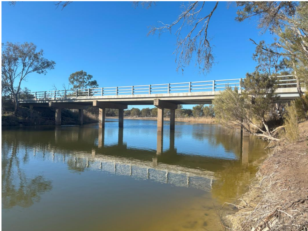
Photograph 21 – Nhill-Jeparit Road bridge.
