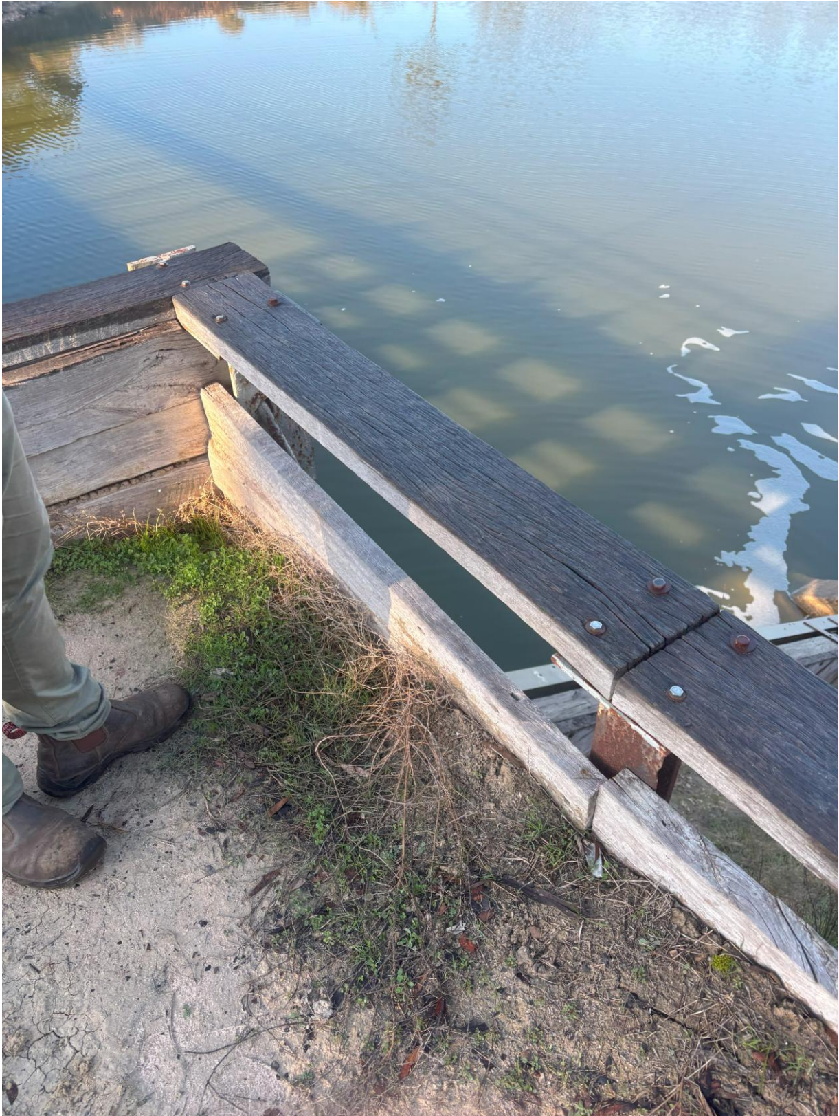
Photograph 13 – Right side retaining wall and abutment.
