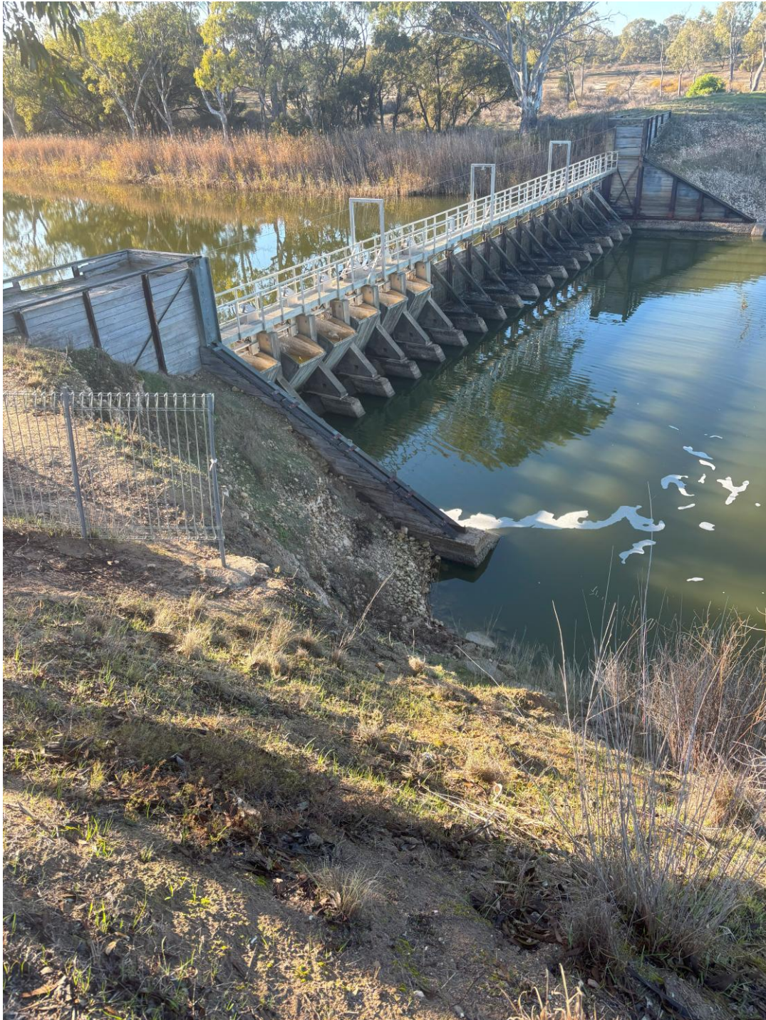
Photograph 8 – Right side abutment downstream of the weir.
