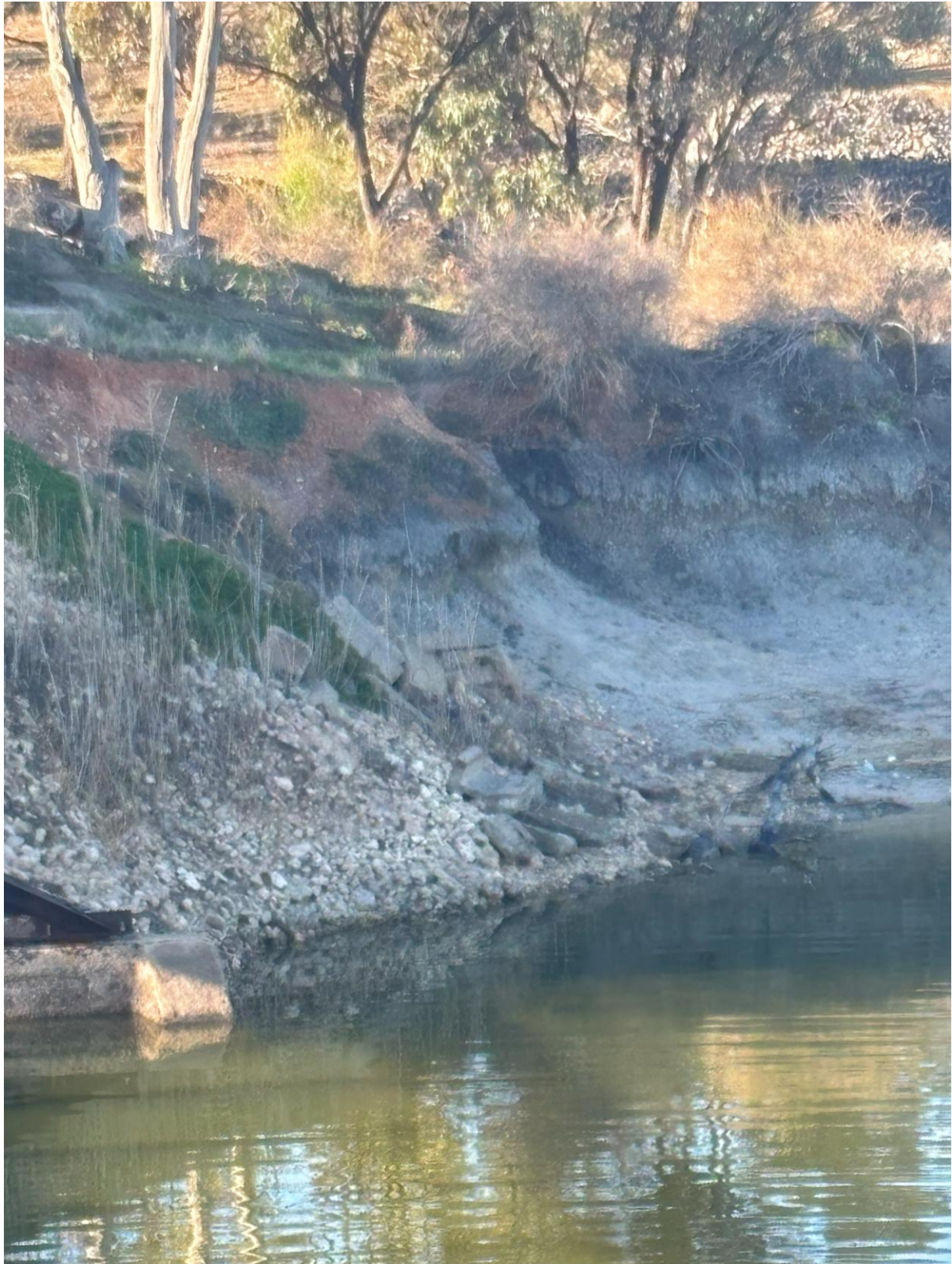
Photograph 16 – Left bank downstream of the weir.
