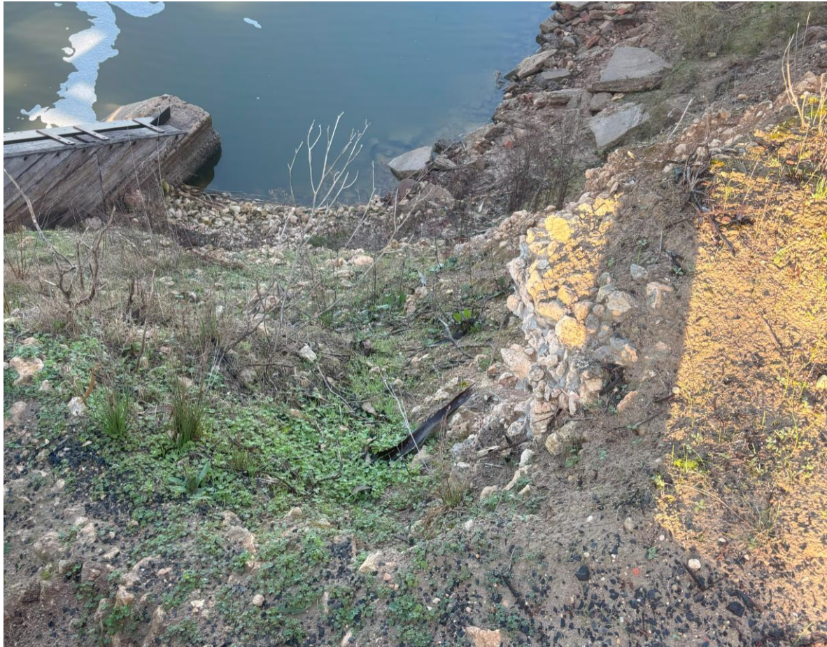
Photograph 4 – Downstream end of the RHS retaining wall.
