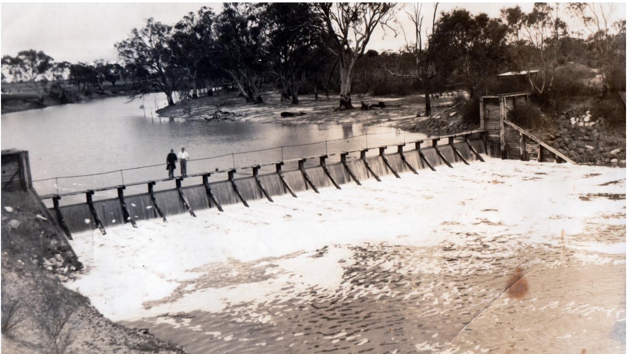
Figure 2-6 Jeparit Weir Photo (Source: Jeparit Historical Society)
