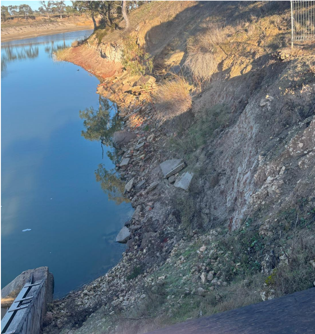
Photograph 3 – Right abutment immediately downstream of the weir.
