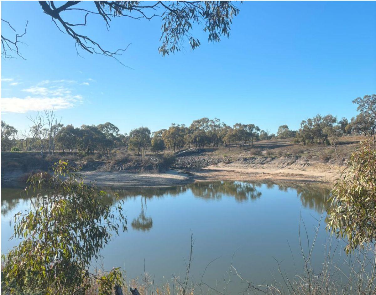
Photograph 6 – Spillway on downstream left side of river.
