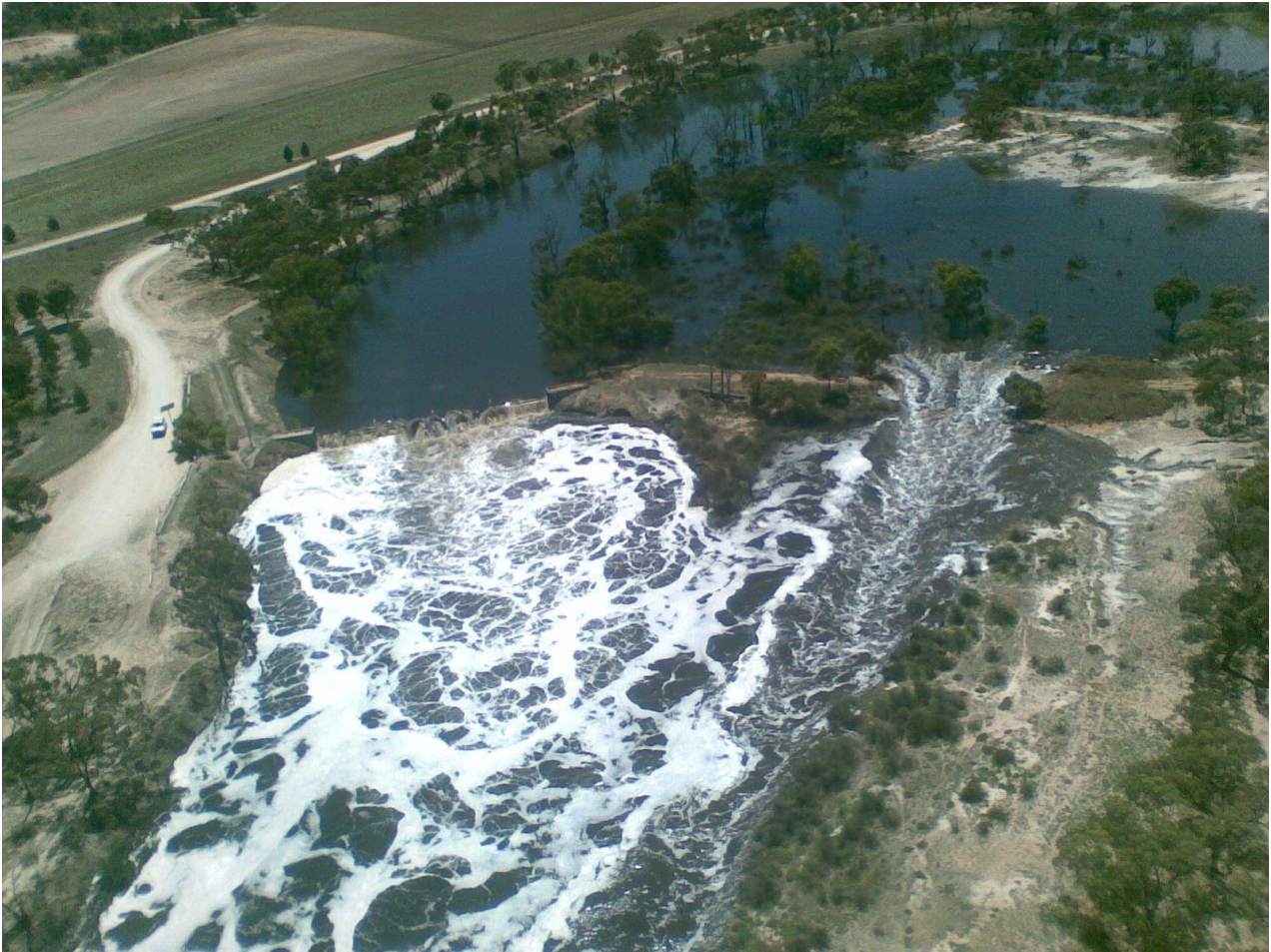
Figure 4-3 Overtopping of the Jeparit weir during the 2011 flood event
