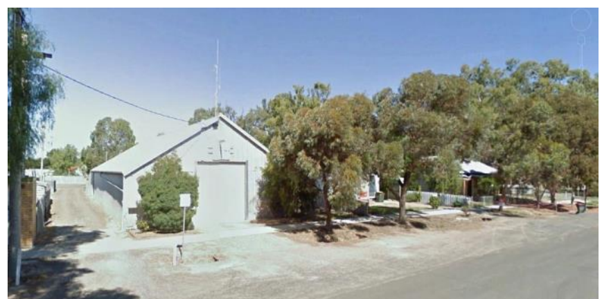
Figure 16 - Current SES building from Lochiel Street
