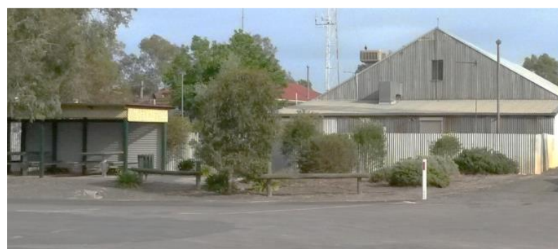
Figure 19 – Open space at rear of current SES building
