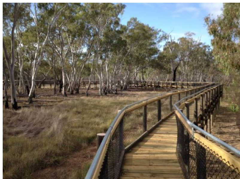
Figure 39 - Nhill Swamp Boardwalk (Source - http://www.mailtimes.com.au/story/3281917/community-unveils-new-boardwalk/ )
