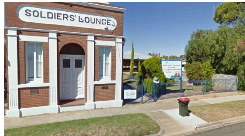
Figure 15 - Current Nhill Kindergarten in Clarence Street
