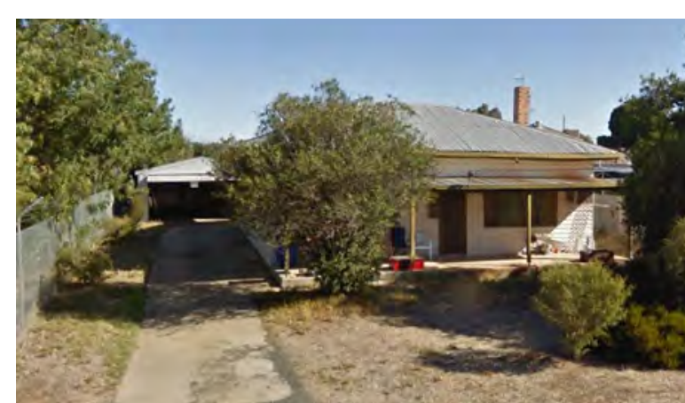
NO. 23 FRASER ST, NHILL (ADJACENT SITE) EXISTING DWELLING, WEATHERBOARD AND TIN ROOF
