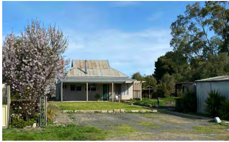
NO. 27 FRASER ST, NHILL (SUBJECT SITE) EXISTING DWELLING, WEATHERBOARD AND TIN ROOF
