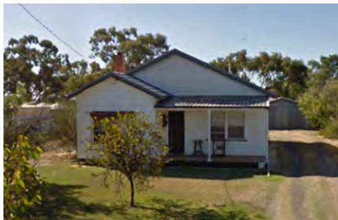
NO. 28 FRASER ST, NHILL (ADJACENT SITE) EXISTING DWELLING, CEMENT SHEET AND TILED ROOF
