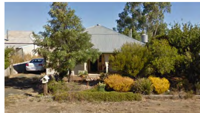
NO. 29 FRASER ST, NHILL (ADJOINING SITE) EXISTING DWELLING, WEATHERBOARD AND TIN ROOF
