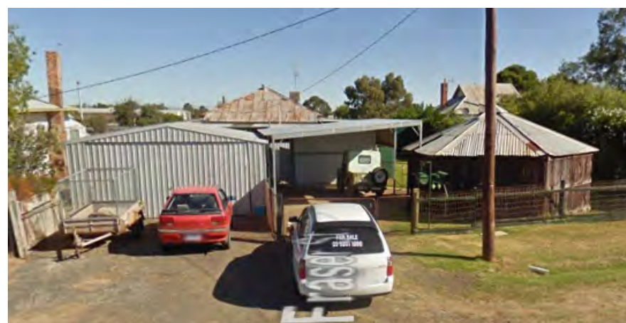
NO. 25 FRASER ST, NHILL (ADJOINING SITE) EXISTING DWELLING, UNKNOWN CLADDING AND TIN ROOF
