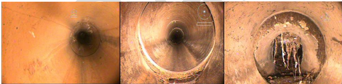
Figure 16 Pipe Condition Example: 2, 5, 8 from left to right
