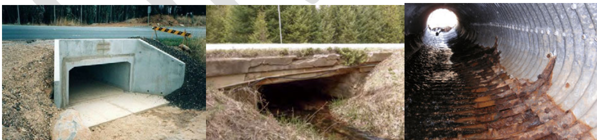
Figure 10 Culverts Condition Example: 1, 5, 7 from left to right
