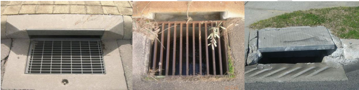
Figure 18 Pit Condition Example: 1, 4, 7 from left to right
