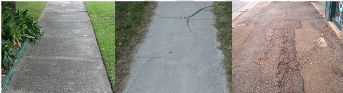
Figure 14 Pathways Condition Example: 4, 6, 9 from left to right
