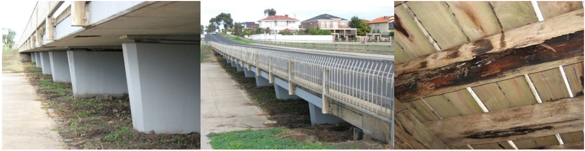
Figure 8 Bridge Condition Example: 1, 4, 9 from left to right
