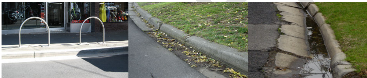
Figure 7 Kerb Condition Example: 1, 5, 9 left to right
