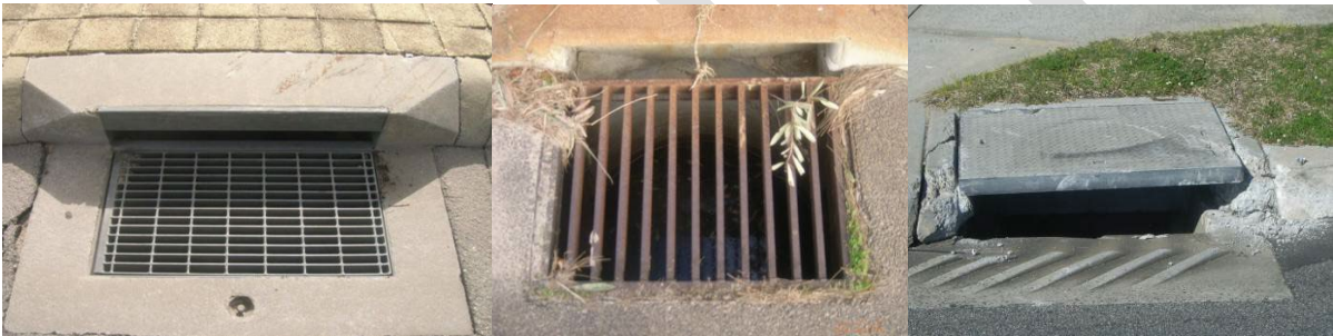
Figure 18 Pit Condition Example: 1, 4, 7 from left to right
