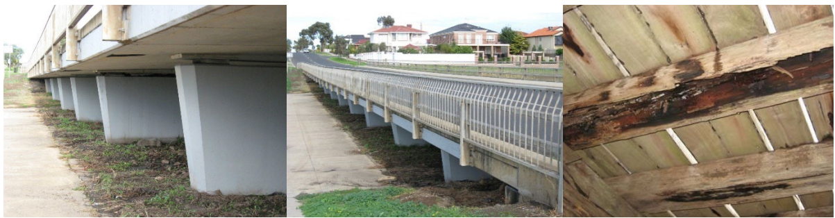
Figure 8 Bridge Condition Example: 1, 4, 9 from left to right
