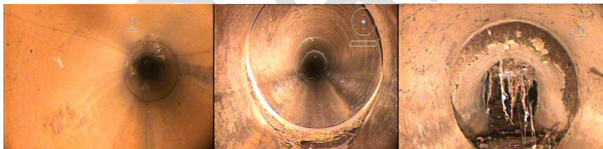
Figure 16 Pipe Condition Example: 2, 5, 8 from left to right
