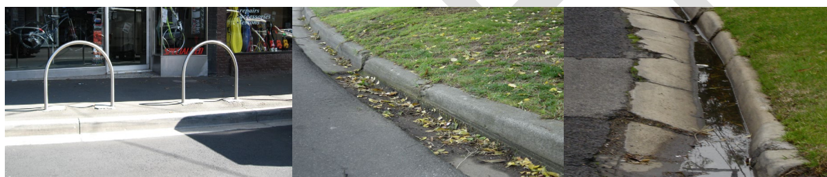
Figure 7 Kerb Condition Example: 1, 5, 9 left to right
