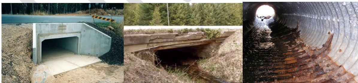
Figure 10 Culverts Condition Example: 1, 5, 7 from left to right
