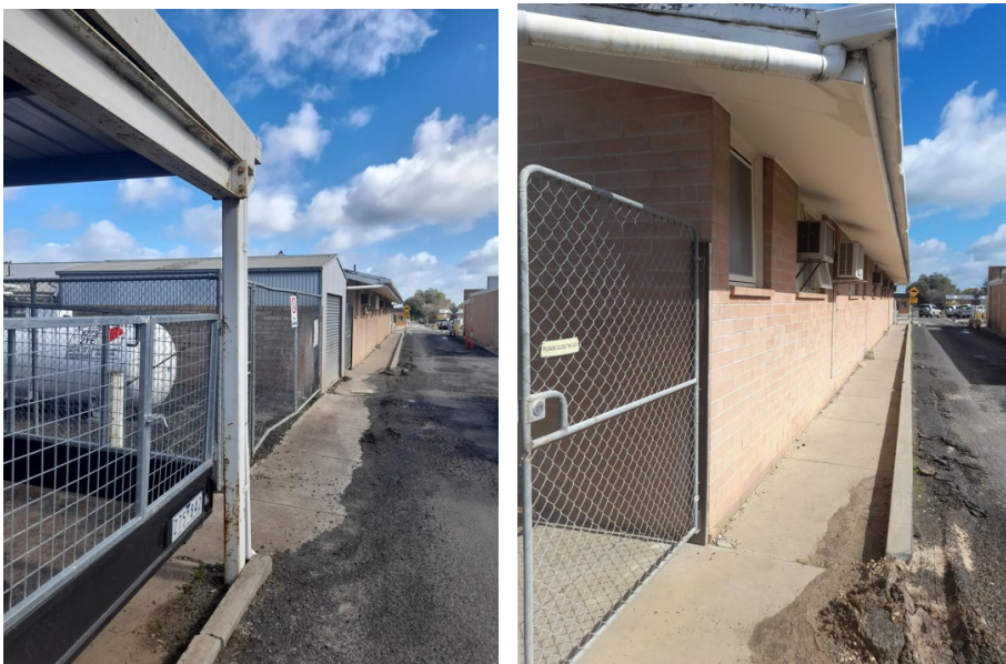
Photos above of rear of site and the footpath that is mostly within the site
