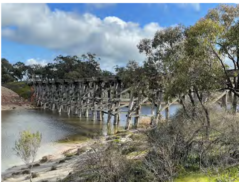
Jeparit Railway Bridge (Wimmera River)
