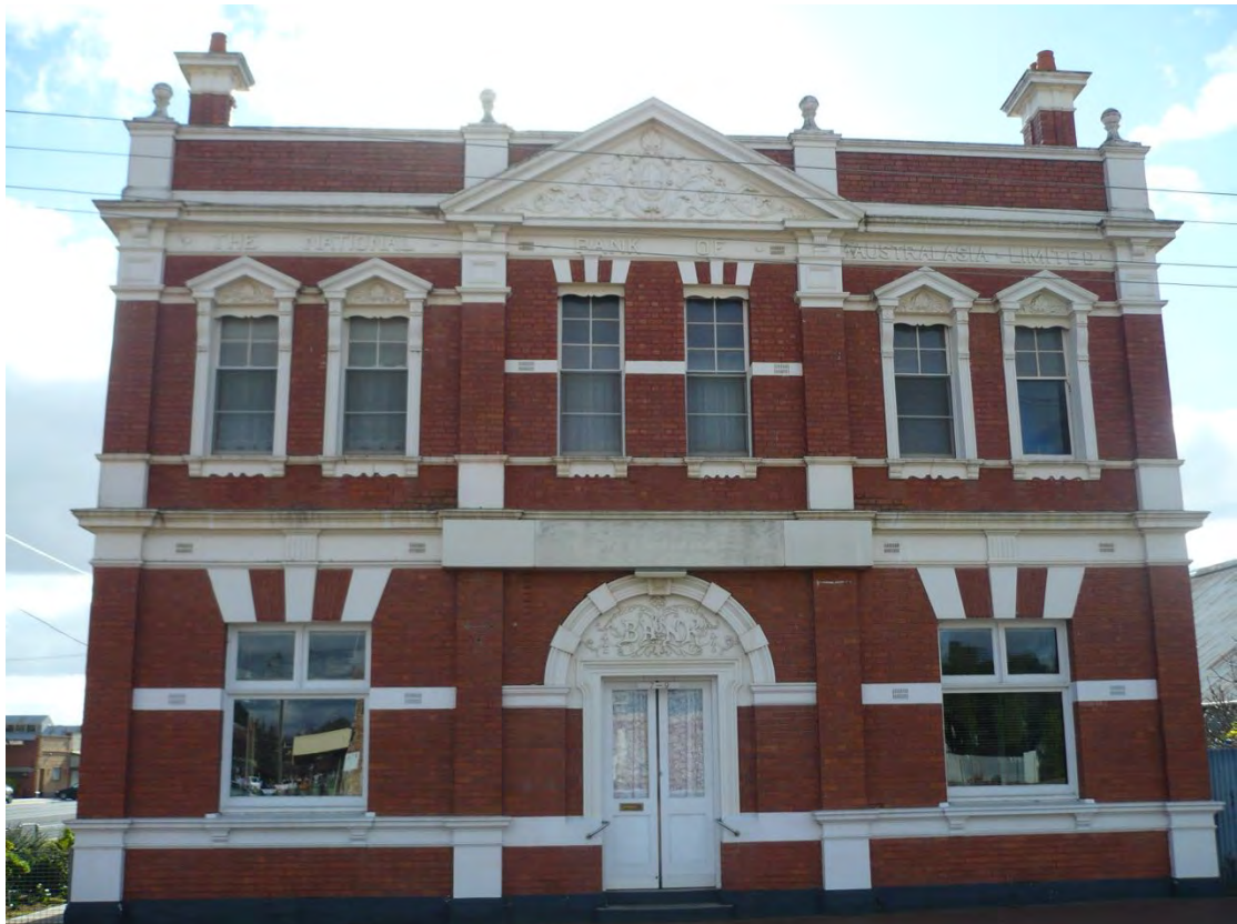
Example 2 - The contrast between the unpainted face brickwork and the painted render is an important feature of this former bank in Lochiel Street, Dimboola.
