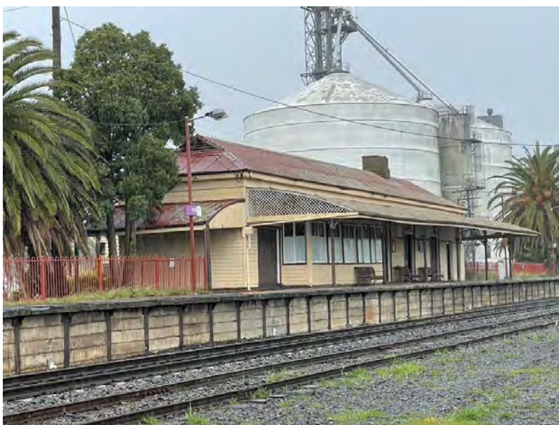
Nhill Railway Station
