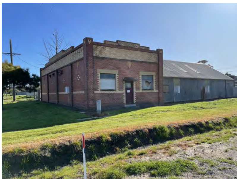
Dimboola Power House
