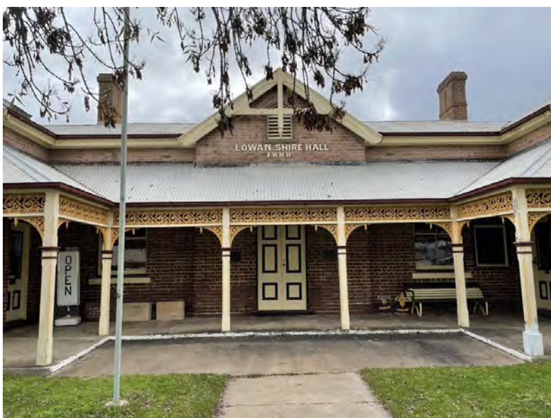
Lowan Shire Hall (Former)
