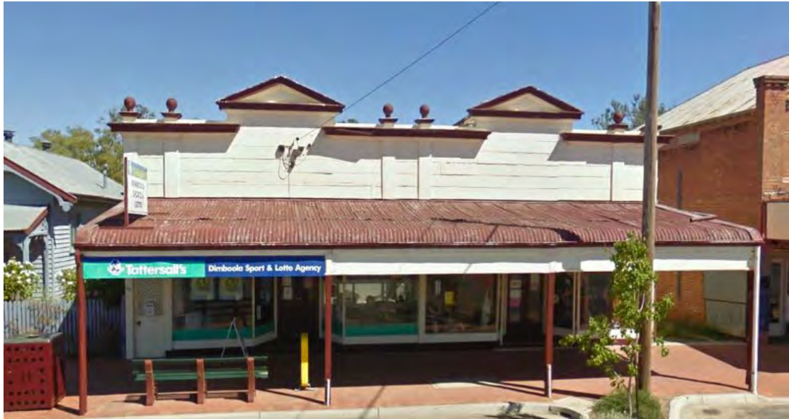
Example 1 – the simple two-colour scheme for this pair of timber shops in Lloyd Street, Dimboola is generally appropriate, although the use of the dark colour to the parapet detail is not historically correct – a deeper shade of the light colour would be better.
