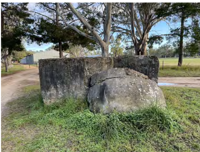
Dimboola Pumping Station site
