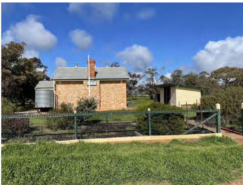
Kenmare Primary School No.3221
