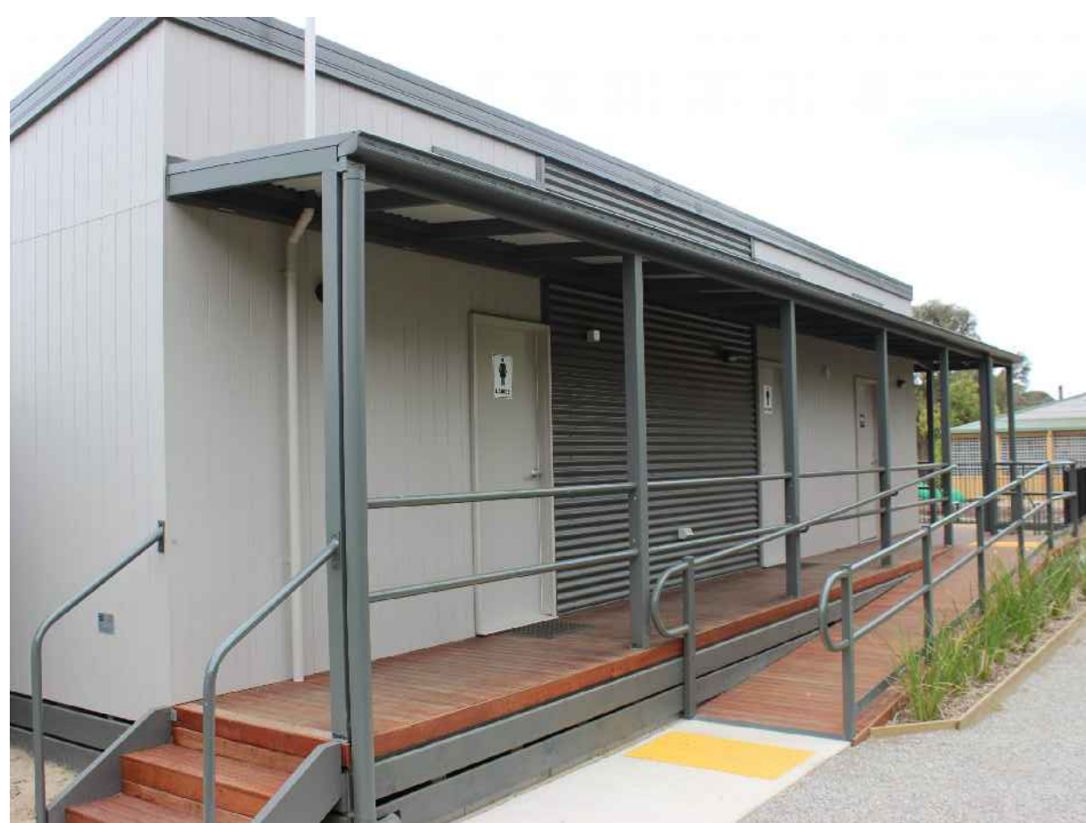
Amenities Block - including all abilities access camp
